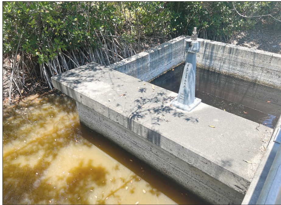
The structure on Tarpon Bay Road that separates the east basin of the Sanibel River (water on the right within concrete enclosure) from the west basin (water outside the enclosure)
